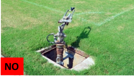
Metal cover too near corner
