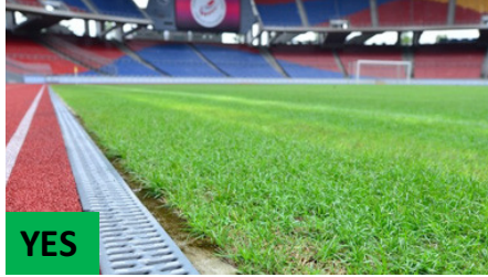
Proper drainage cover
